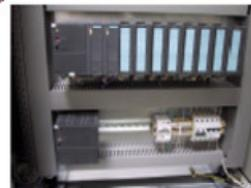
PLC control cabinets based on Simatic CPU414 & ET200M
