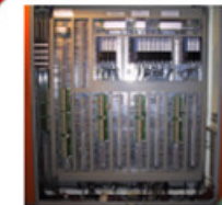
PLC control cabinets
